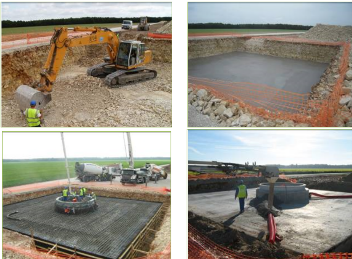
Figure 16: chantier fondation - source Siemens Gamesa
